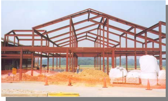
Arnold Palmer Regional Airport Terminal Building Construction
