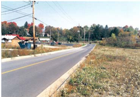
Local Road Project – Meadow Lane City of DuBois, PA – constructed 1997/98
