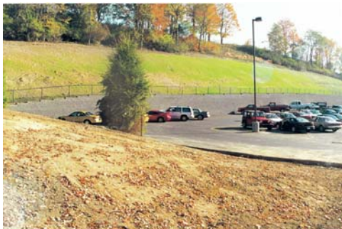
Pennsylvania State University-DuBois Campus Parking Lot – constructed 2000
