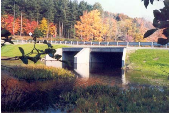
DuBois Reservoir Bridge Union Twp., Clearfield Co., PA
