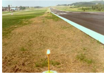
Arnold Palmer Regional Airport Runway Lighting Westmoreland County, PA
