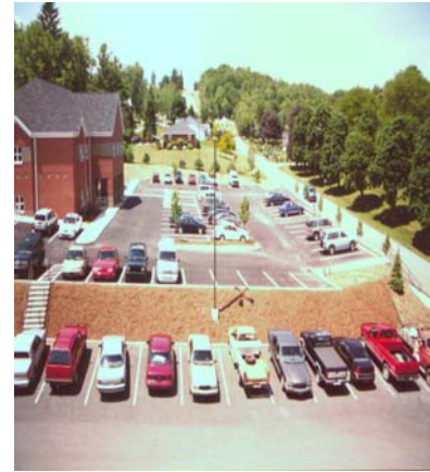
DuBois Regional Medical Center Parking Lot Lighting
